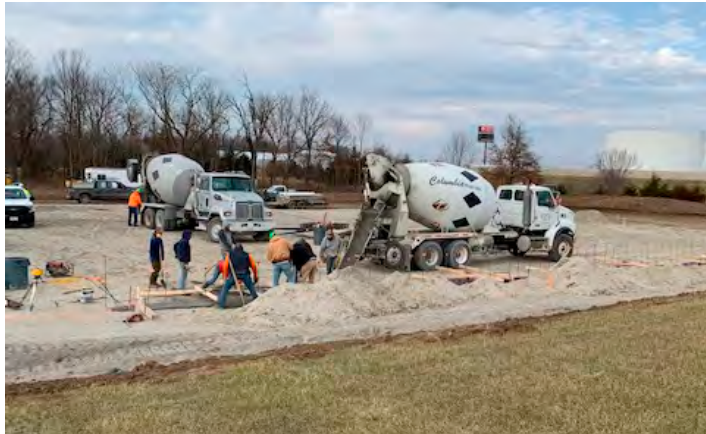
December 27th, concrete footings are poured.
