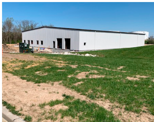
South side and view of docks
