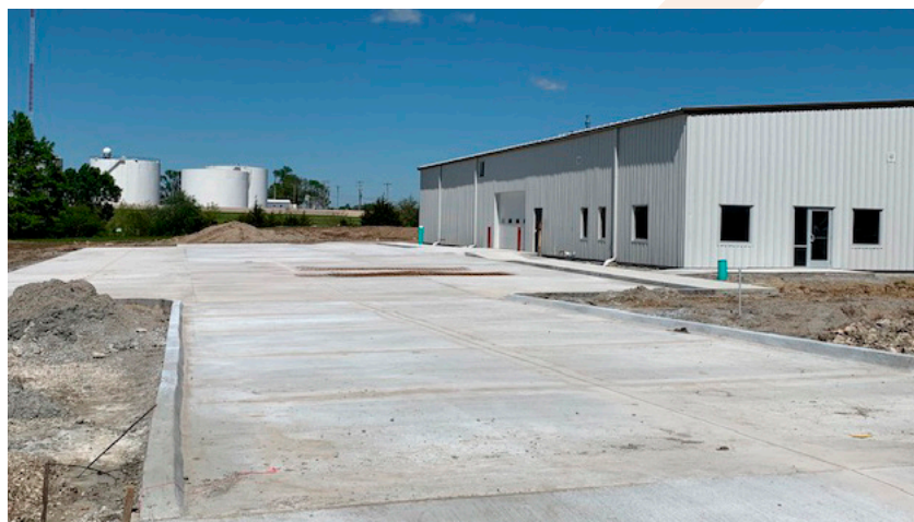
North side with concrete lot and drive
